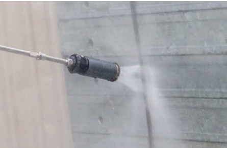
Cleaning of shuttering and scaffolding
