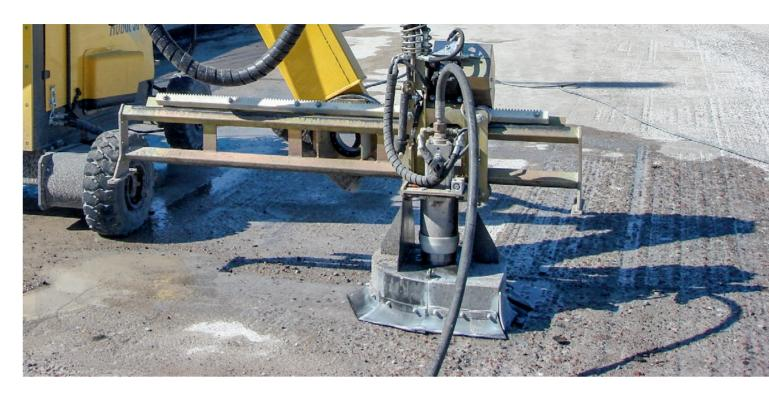
Hammelmann high pressure units offer a wide performance range, for hand-lancing operation and up to heavy concrete removal with robots.
